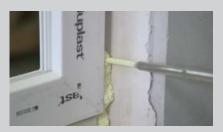
DuPont<sup>™</sup> Insta Stik<sup>™</sup> Flex+ is a moisture-curing, fire-resistant, single-component polyurethane foam. It is mainly used for the permanent, airtight installation of windows and doors.
