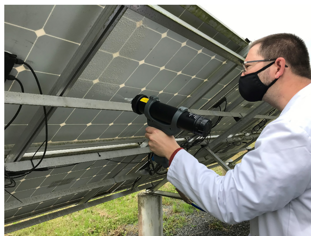
FIGURE 13 Application of flowable silicone sealant without module dismounting by spraying
